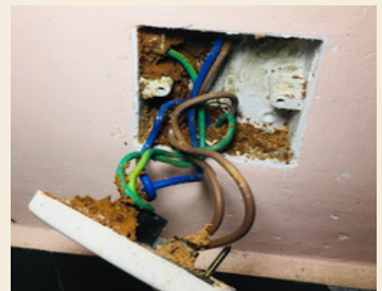
Figure 10.0: This figure shows the damage caused by ants
