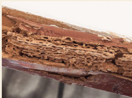
Figure 6.0: This figure shows that the wooden structure has been damaged caused by termites
